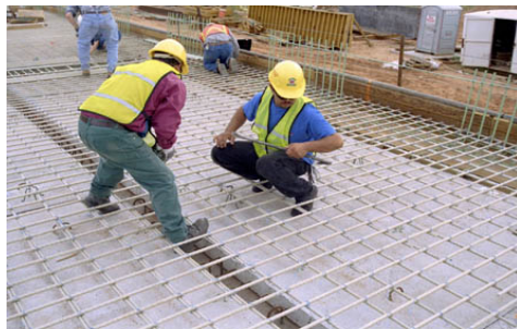
Fig. 2. – Bridge deck reinforced with FRP bars
