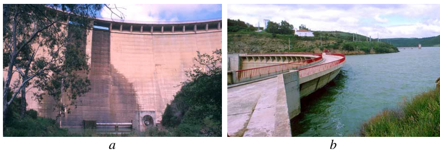
Fig. 7. – Prototype Arch Dam - Odiaxere Dam from Portugal; a – downstream view; b – upstream view.
