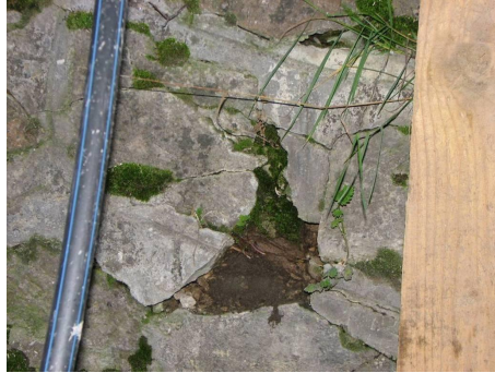
Fig. 7. – Portions of the wall with extended cracks, detachments of stone and abundant vegetation.
