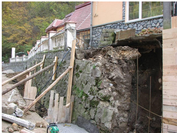
Fig. 8. – Blocking the movement of the retaining wall (using concrete works) and sustaining its wall parament.
