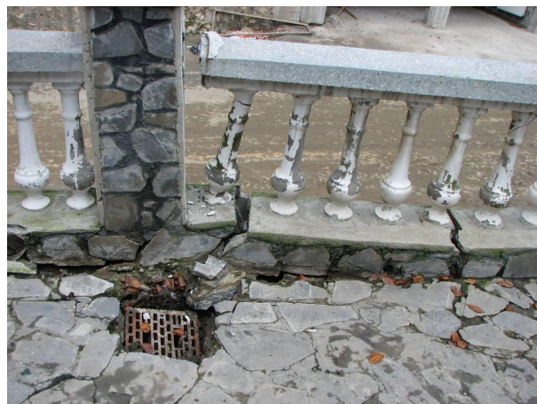
Fig. 4. – Cracks in the protection bulwark area.
