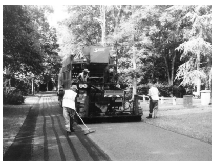
Fig. 1. – Coloured asphalt laying.
