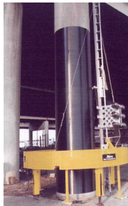
Fig. 6 – Automated RC column wrapping.
