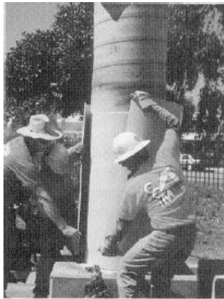
Fig. 5 – Confining system based on prefabricated FRP elements.
