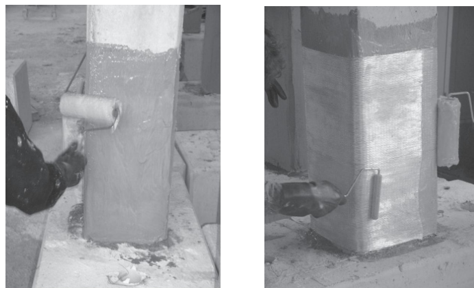
Fig. 4 – Wet lay-up confining system.
