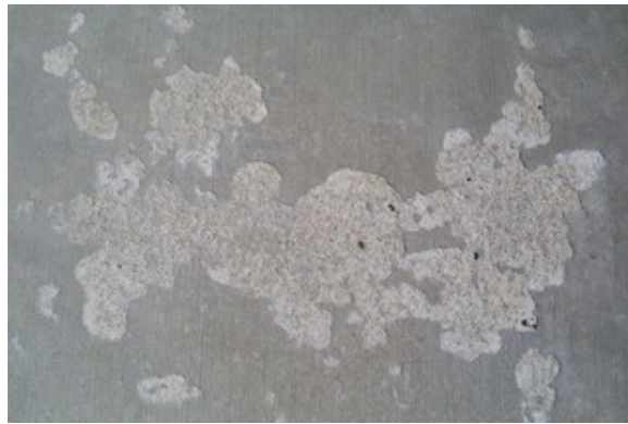
Fig. 4 – Spalling and scaling of the surface.
