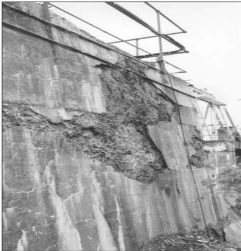
Fig. 7 – Damages of concrete caused by freeze–thaw.
