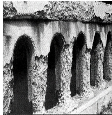
Fig. 7 – Damages of concrete caused by freeze–thaw.
