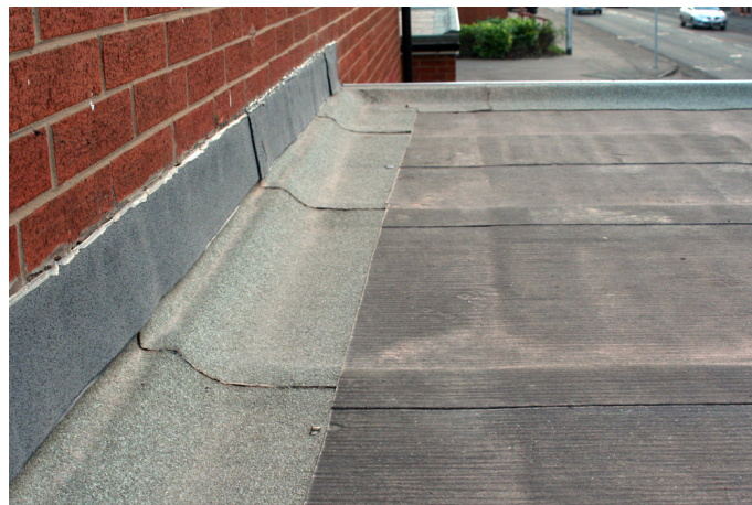
Fig.9 – Flat roof cover with bituminous membrane.
