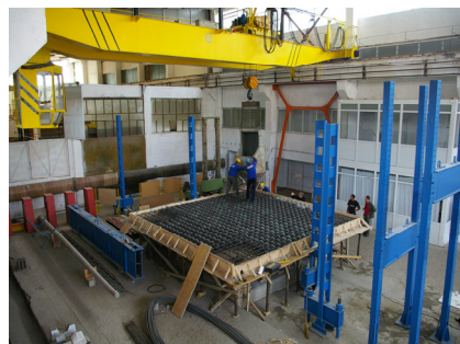
Fig. 8 – General view during pouring.
