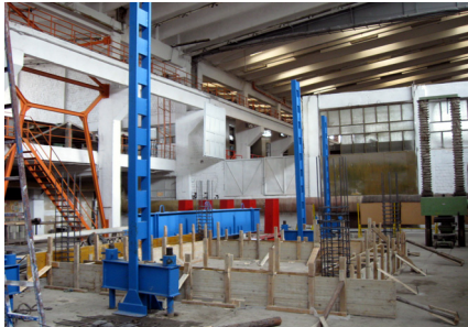
Fig. 5 – Connection beams formwork.
