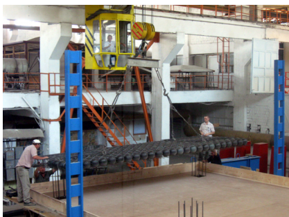
Fig. 7 – Mounting of Bubble Deck modules.
