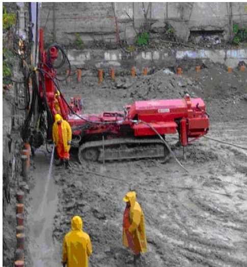
Fig.4 – Execution of pilots using the jet grouting method.
