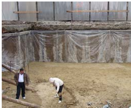
Fig. 3 – Jet grouting at Lascar Hotel, Bucharest, Romania [7].
