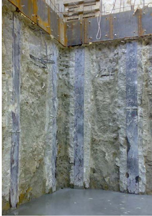
Fig.5 – Columns realized using the jet grouting method.
