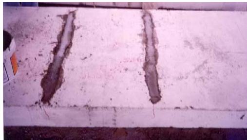
Fig.2 – Cracks repaired using grout pouring technique.
