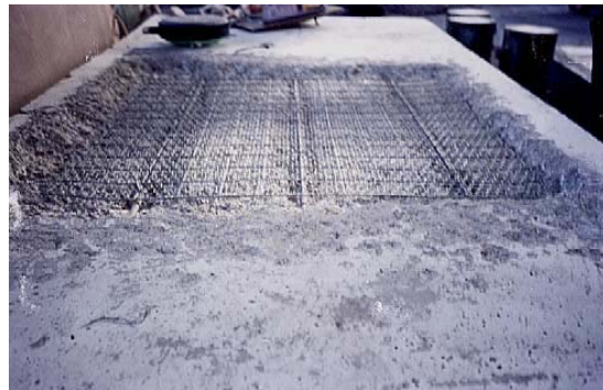
Fig.4 b – Wired mesh used for repair.
