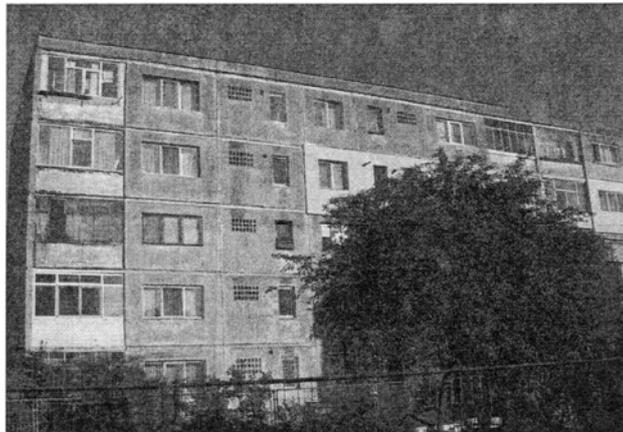
Fig. 1 – A P+4 concrete panels building from Iași city.
