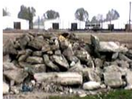
Fig. 3 – Debris resulting from demolition.
