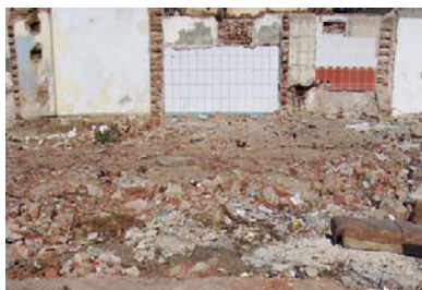
Fig.4 – Structure during demolition.
