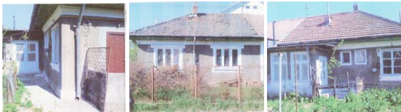
Fig. 1 – Existing structure before demolition.
