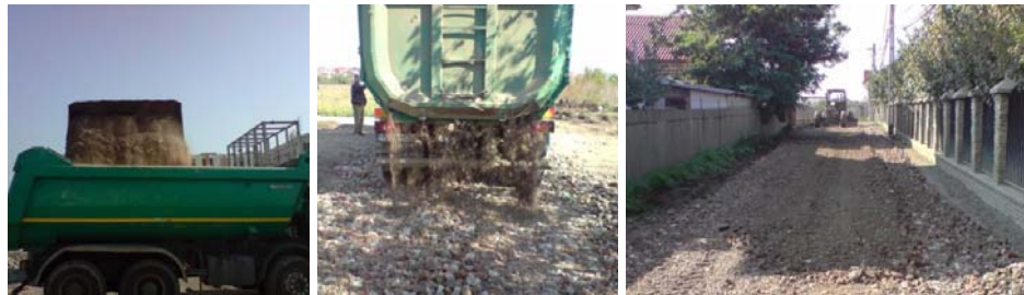
Fig. 5 –Use of crushed mixture from demolition sites in earthworks applications.
