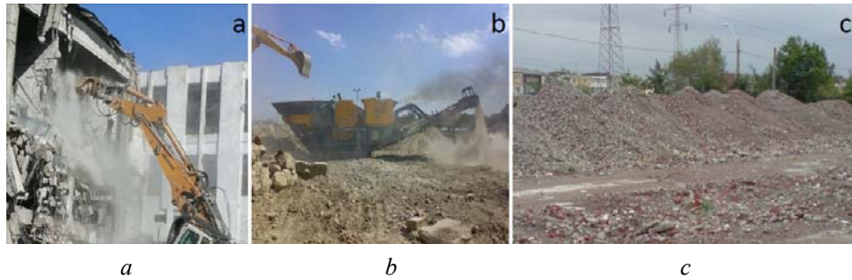
Fig. 4 – Demolition process and crushing of demolished material.
