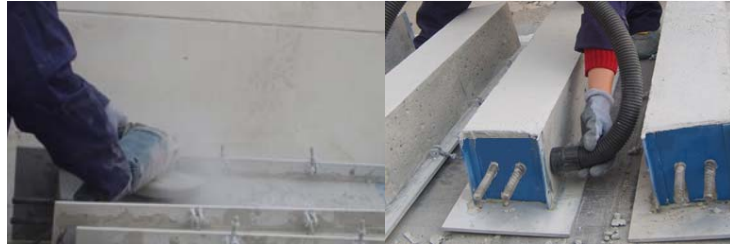
Fig. 3 – Preparation of the concrete surface.
