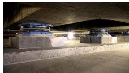
Fig. 4 – Friction pendulum system.
