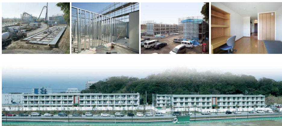
Fig. 3 – Nittetsu Super Frame, Kitakyushu Science and Research Park during erection and finished.
