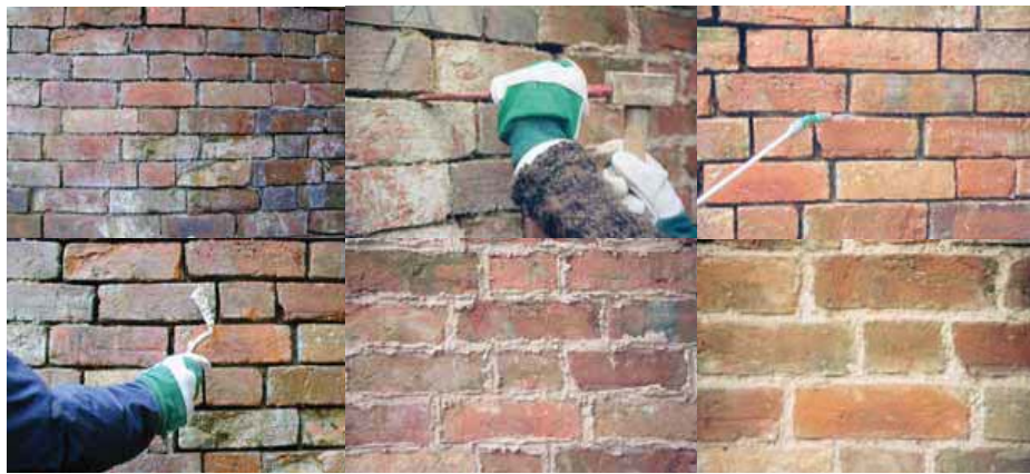
Fig. 2 – Steps for repointing strengthening intervention.
