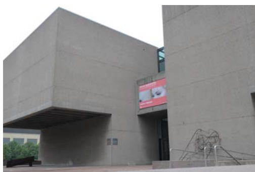
Fig. 1 – Exposed concrete facade - Everson Museum of Art, Syracuse, New York.
