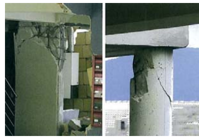
Fig.3 – Formation of the plastic articulation in the pilots.
