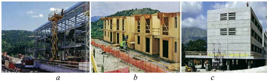
Fig. 7 – Types of structures: a – metal superstructure; b – wood superstructure; c – concrete superstructure.
