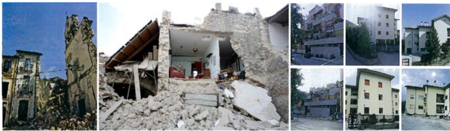
Fig. 4 – Masonry structure damage.
