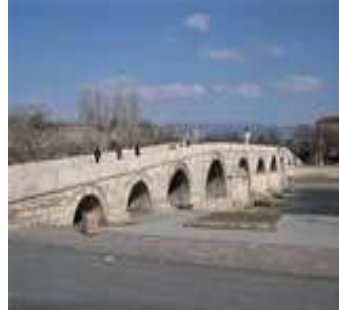
Fig. 3 – Stone bridge from South of France.
