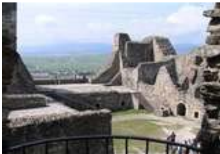
Fig.6 – Neamț Fortress (restored).
