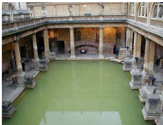
Fig. 1 – Public bath built on foundations of adjoining Roman, Bath, England.
