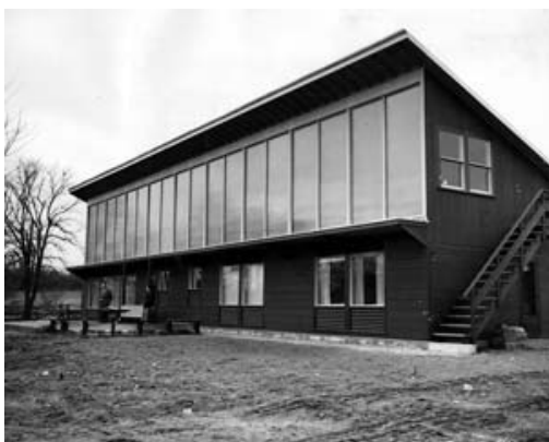
Fig. 3 – Telkes Mária house – Dover, Boston.
