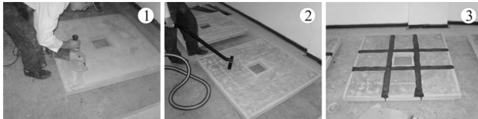
Fig. 3 – Substrate preparation: 1 – removing cement laitance and traces of form-release oil; 2 – vacuum dust removing; 3 – marking and applying the primer.
