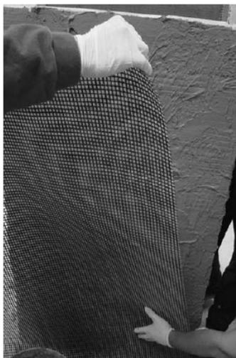
Fig. 1 – Reinforcing masonry by textile embedded in cementitious mortar (Papanicolaou *et al.*, 2008).
