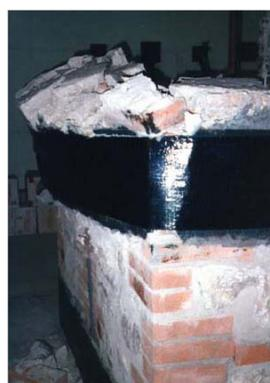
Fig. 4 – Fiber wrapping/encasement of masonry buildings in FRP shells (Borri *et al.*, 2003).
