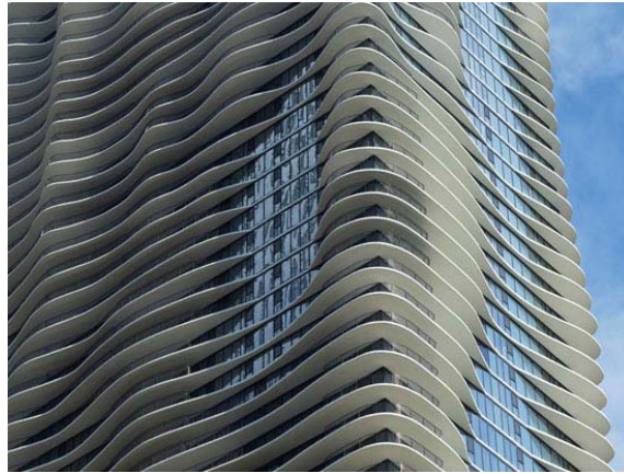
Fig. 1 – Skyscraper with a solar shading system to prevent unnecessary heat gain.
