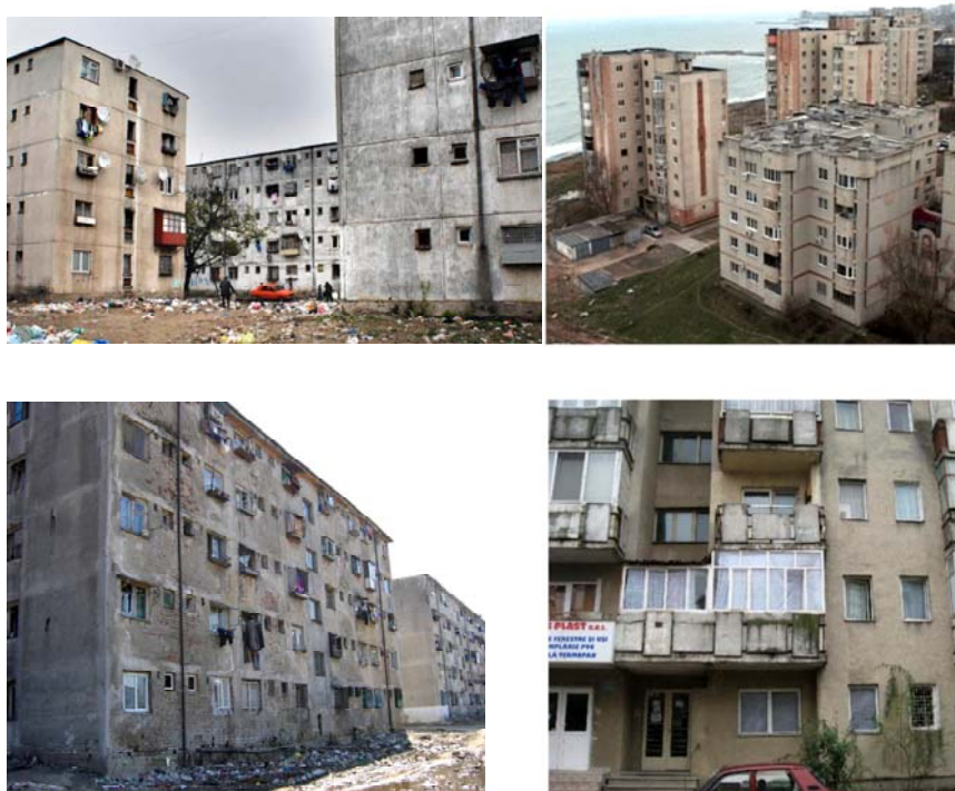
Fig. 3 – Damages caused by moisture (infiltrations and condensed water) may have major impact on the building's structure and especially on the quality of the living space.
