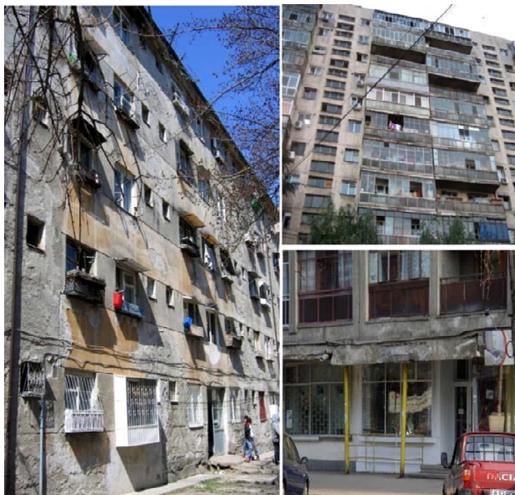
Fig. 2 – Different types of degradation on different levels (structural, finishings, etc.).
