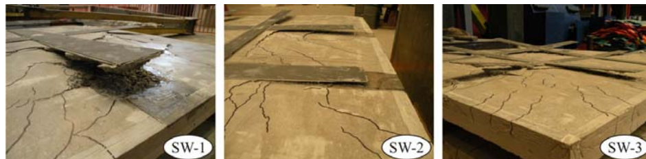
Fig. 3 – Bond failure of the strengthening system.
