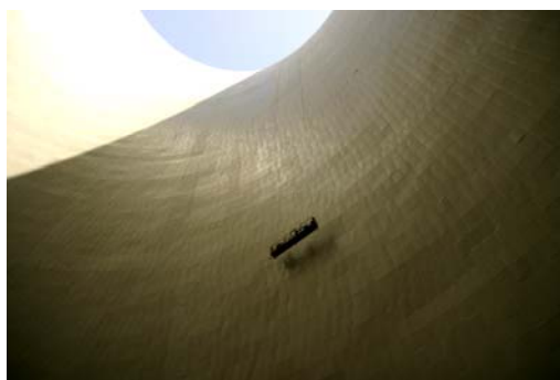
Fig. 1 – Work platform in a natural draught cooling tower.
