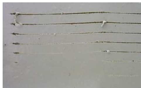
Fig. 3 – Failed attempt with a multi-cutter tool.
