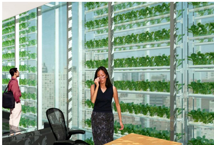
Fig. 2 – Image of vegetable garden integrated in a vertically double glazed façade structure of an office building ( www.mediaderive.blogspot.ro/2010/07/terraform-1-workshop-part-2-building.html ).
