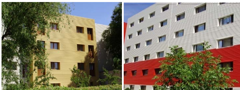
Fig. 1 – Ventilated facades made of corrugated metal sheets used for the thermal rehabilitation of students' halls in "Tudor Vladimirescu" campus, Iași.
