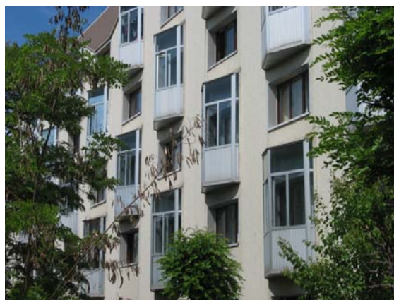
Fig. 2 – Thermal rehabilitation of the T14 student hall.
