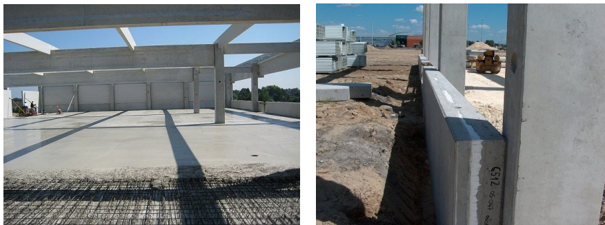
Fig. 1 – Slab-on-ground industrial floor and footing wall panel perimeter insulation.
