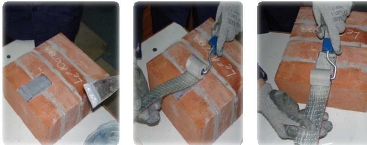
Fig. 2 – Applying the FRP strips on the masonry substrate.
