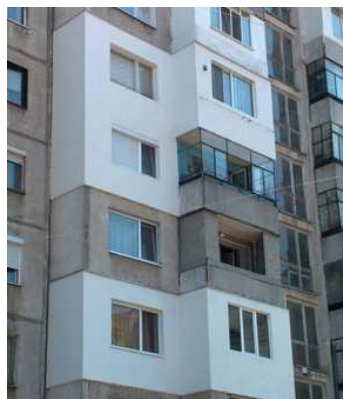
Fig. 6 – Façade partial insulated.
