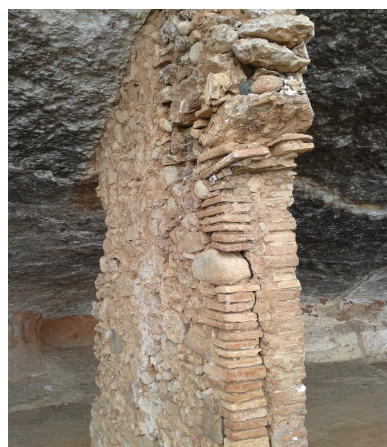
Fig. 2 – Mortar without continuity caused by aggressive environment's agents, XV th century masonry.
