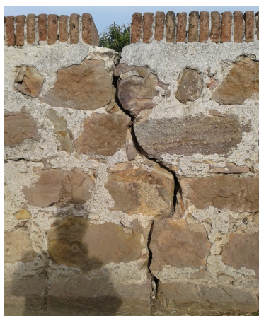
Fig. 1 – Damaged masonry joints caused by water infiltration, XVII th century masonry.
