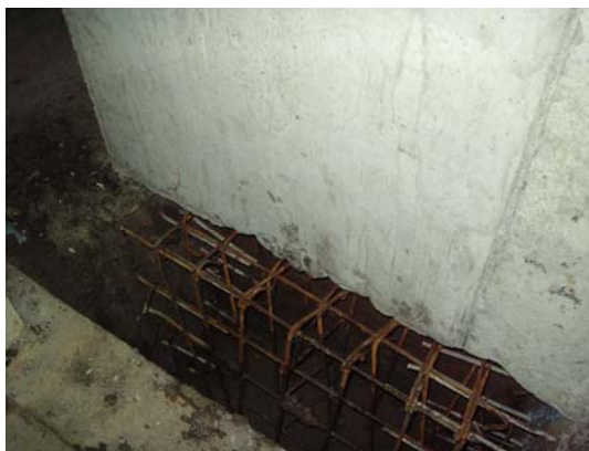
Fig. 8 – Foundation reinforcement during execution.
