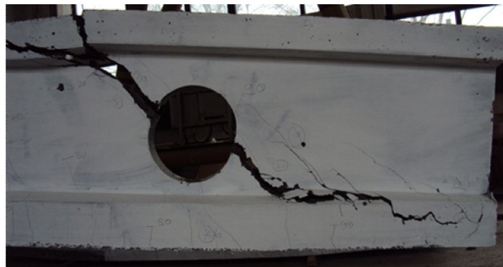
Fig. 4 – FOD beam after failure.
