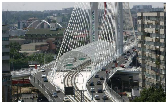
Fig. 2 – Basarab Overpass Bridge, Bucharest, Romania ( http://www.google.ro/imgres?imgurl=http://www.evz.ro/uploads/06basarab_V... ).
