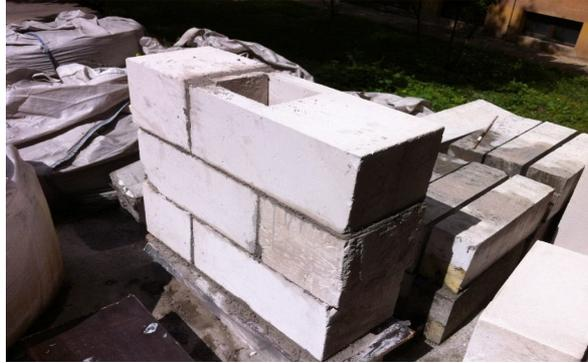
Fig. 6 – Building the vertical hollow masonry section.
