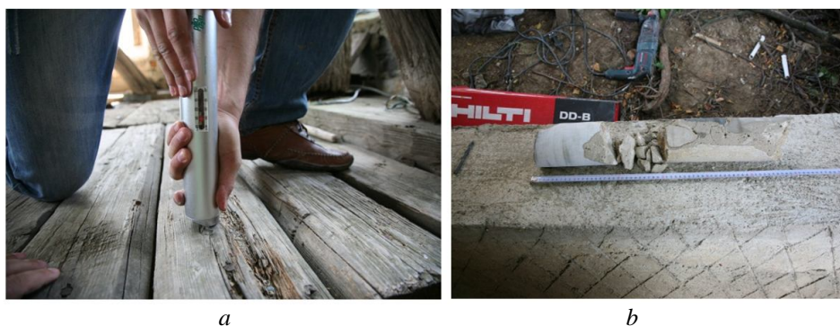
Fig. 2 – On site investigation on St. Simion Tower: a – testing wooden elements with Pilodyn sclerometer; b – extracted mortar and stone specimen by core boring.
