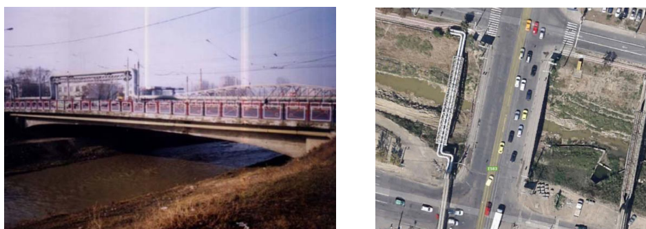
Fig. 1 – RC Bridge location in Iași Tudor Vladimirescu residential neighborhood.
