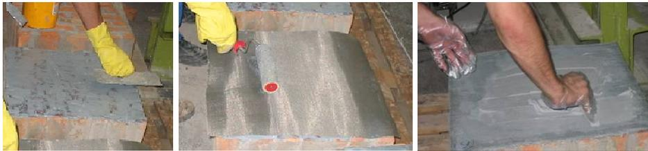
Fig. 1 – Retrofitting solution based on epoxy-glued steel wire mesh (SWM).
