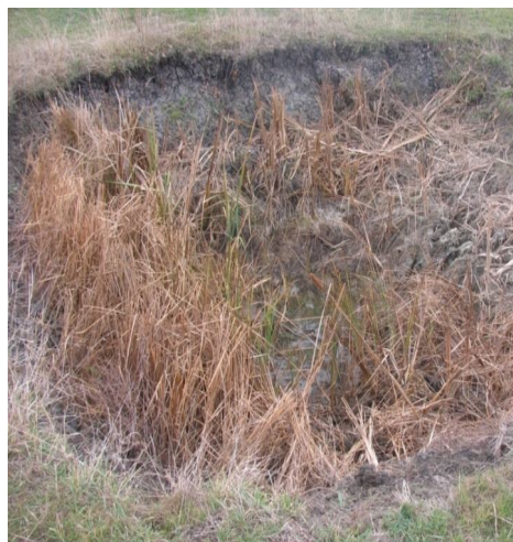
Fig. 2 – Clogged soil profile, with the presence of groundwater to surface.
