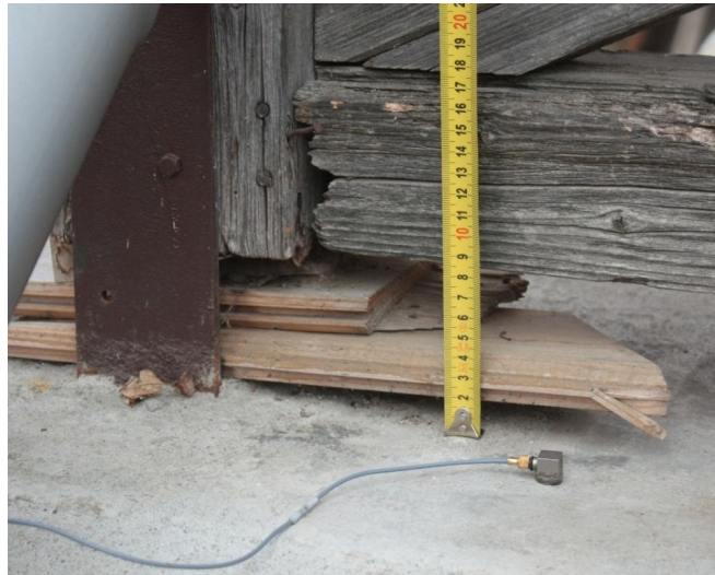
Fig. 5 a – Settlements in column foundations.
