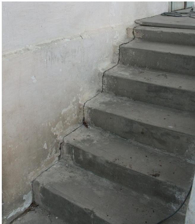
Fig. 5 c – Cracks occurring in the flight of stair ramp
