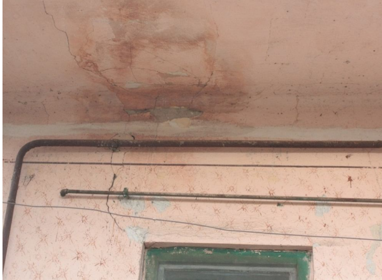
Fig. 5 b – Cracks occurring in the structure.
