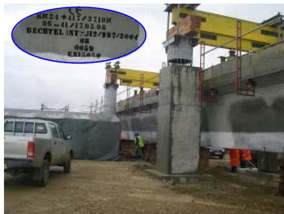
Fig. 2 – The 37.10 m Box Beam on the stand (Mircea *et al.*, 2009).
