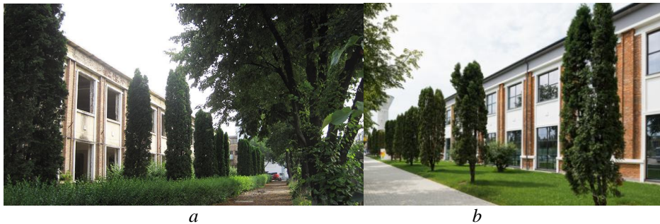
Fig. 10 – a – Building before; b – after reconversion.
