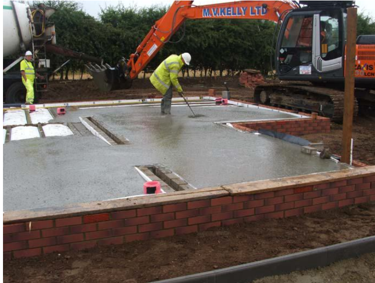
Fig. 3 – Placing slab of SCC (Gaimster & Foord, 2008).
