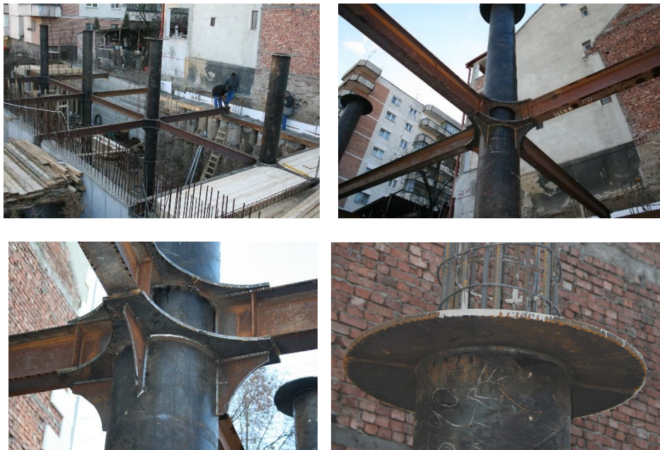
Fig. 3 – Construction S+D+P+3E in Cluj-Napoca (execution phase), (XC Project, 2011).
