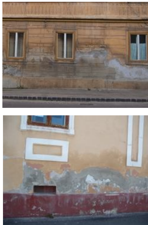
Fig. 2 – Moisture coming from the capillary rise of water in the building elements (Zaharea, 2011).
