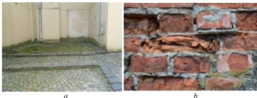
Fig. 14 – a – Building exposed to biological attack; b – Masonry affected by the presence of microorganisms (Strzysewska et al. , 2015).
