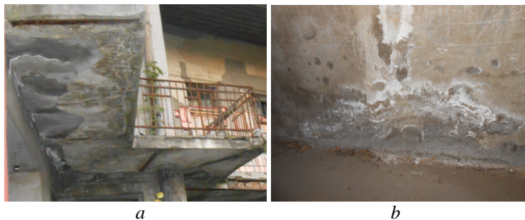
Fig. 18 – a – Efflorescences at the soffit of the exterior slab; b – base area affected by the presence of efflorescences.
