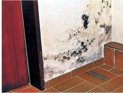
Fig. 3 – Moisture from condensation (Zaharea, 2011).
