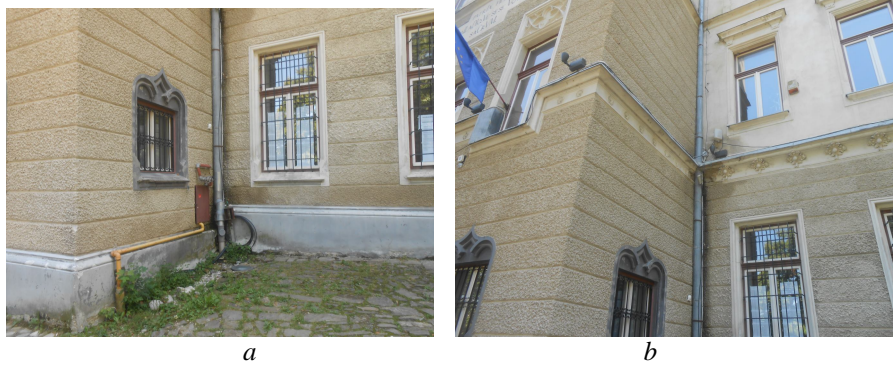
Fig. 1 – a – Lack of vertical systematization; b – damage to the collecting rainwater elements.
