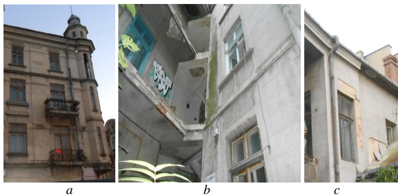
Fig. 16 – a – Kieser Building; b – areas affected by biological attack; c – peeled coating.
