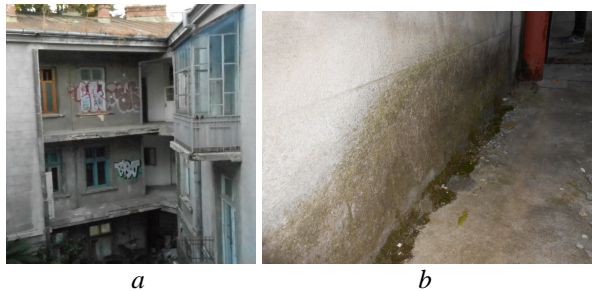
Fig. 17 – a – Defective rainwater collection systems; b – base area affected by the presence of microorganisms.
