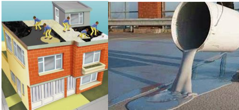
Fig. 5 – Sikalastic-614 waterproof ( http://sporulcasei.ro/hidroizolarea-teraselor... ).
