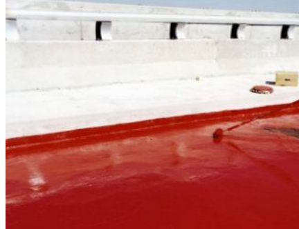
Fig. 6 – Liquid polyurethane membrane.
