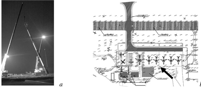
Fig. 1 – *a* – Erection of a 30 m high lighting mast at Iași Airport; *b* – Map showing the extension and modernisation works at the Iași Airport.
