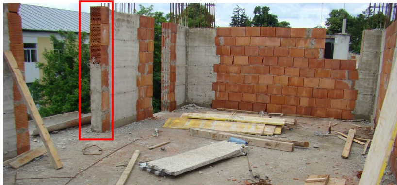
Fig. 1 – On site error due to unqualified workforce.
