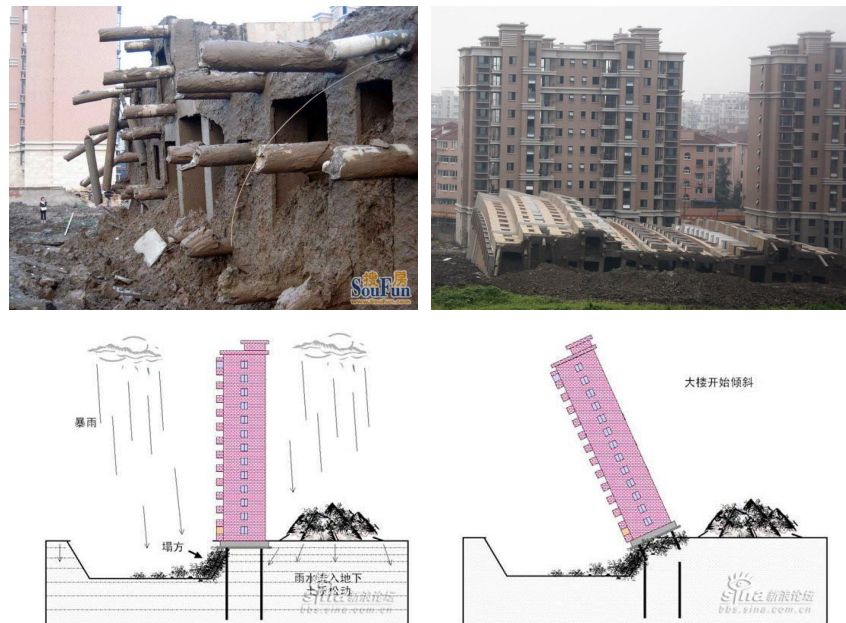
Fig. 4 – Collapse building due to construction error (http://hoax-slayer.com/13-story-building-collapse-china.shtml).
