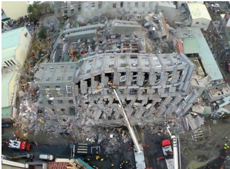
Fig. 5 – Collapse building in Taiwan, 2016.
